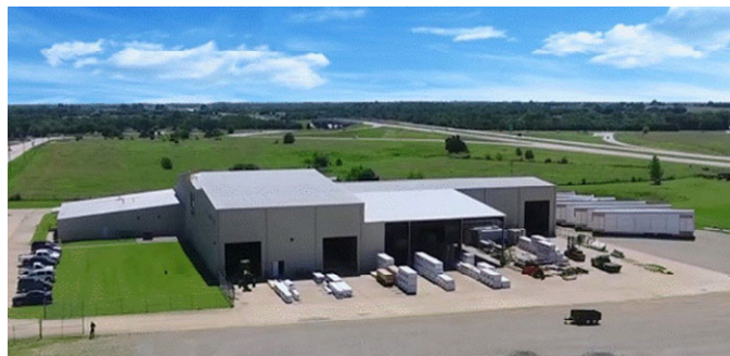
Figure 21 ECHO MODULAR FABRICATION FACILITY
